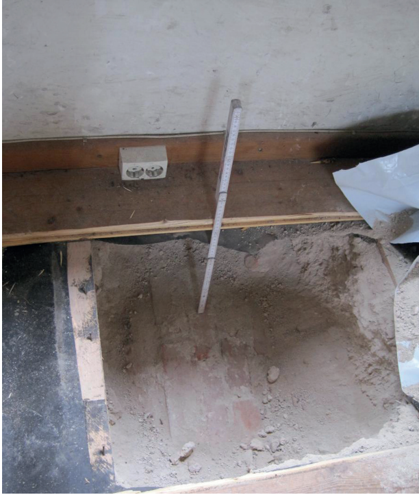
Fig. 6. Photo of a small excavation trench below the pavilion's floor showing parts of the vaulted cellar roof. The folding ruler shows the estimated depth below the modern floor (Photo: Prof. Dr. Dr. von Wachter).
