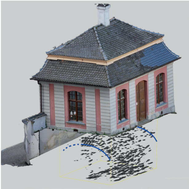
Fig. 11. Photogrammetric 2.5D model of the Baroque garden pavilion with isosurface rendering of the detected barrel vault displayed underneath. The blue lines illustrate the position of the bricked vault.
